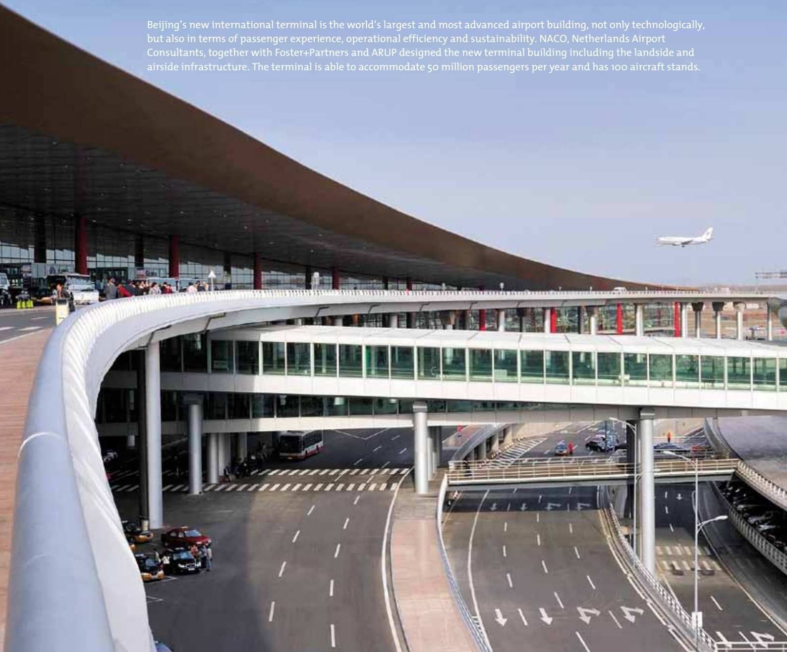
Beijing Capital International Airport Terminal Building 3, China
