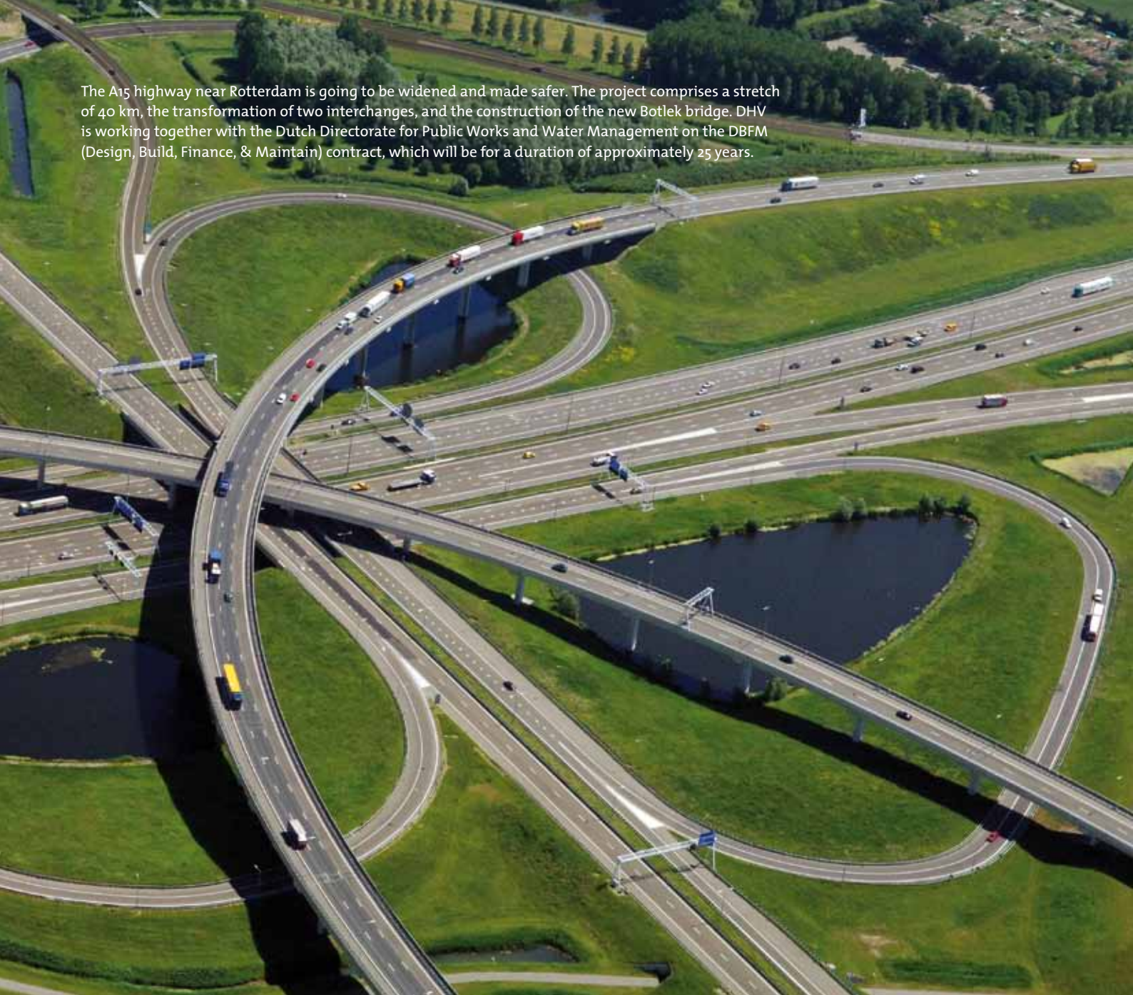
Preparation and tendering of A15, Rotterdam, the Netherlands
