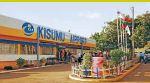
Upgrading Kisumu Airport, Kenya
