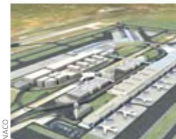
Athens International Airport
