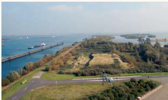
DHV is inspecting 100 kilometers of dikes and 20 civil engineering works in the Volkerak Lake.
