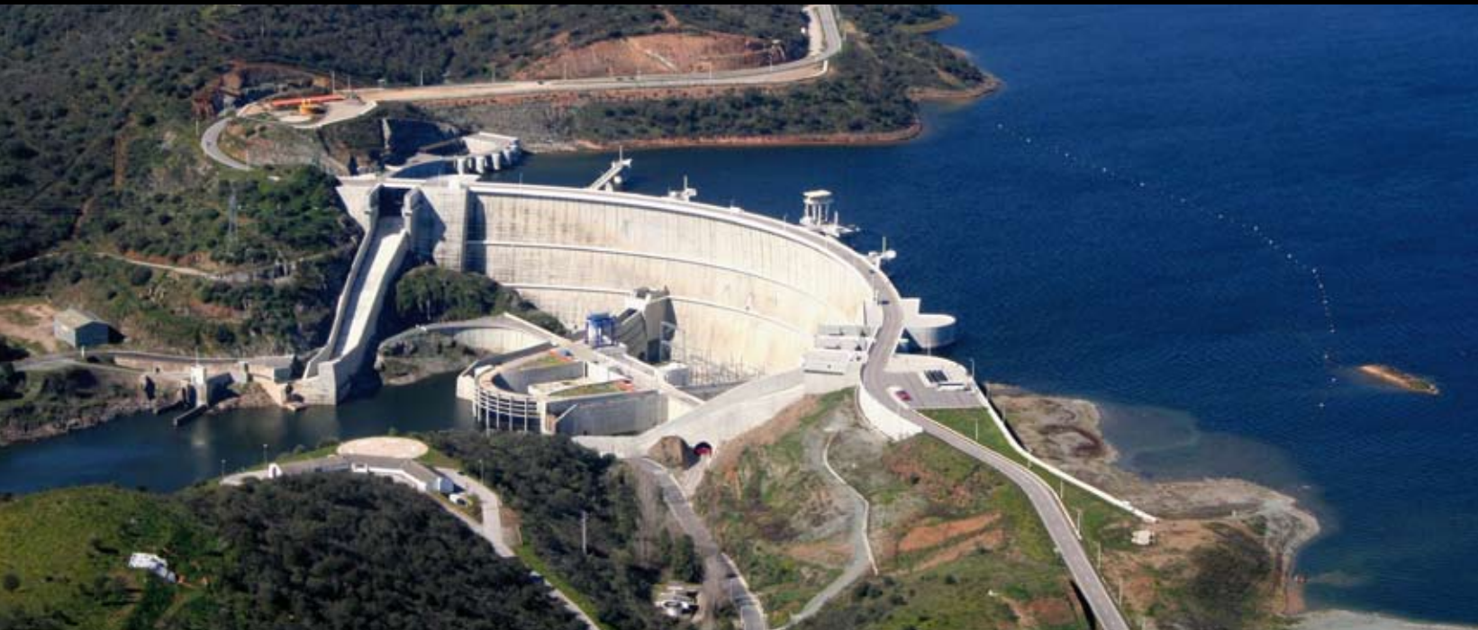
DHV S.A. provides services for the Alqueva Dam Power Reinforcement Project.
