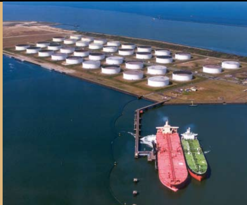
DHV Asset Management will draw up a ten-year maintenance plan for the Maasvlakte Oil Terminal (MOT) in Rotterdam.
