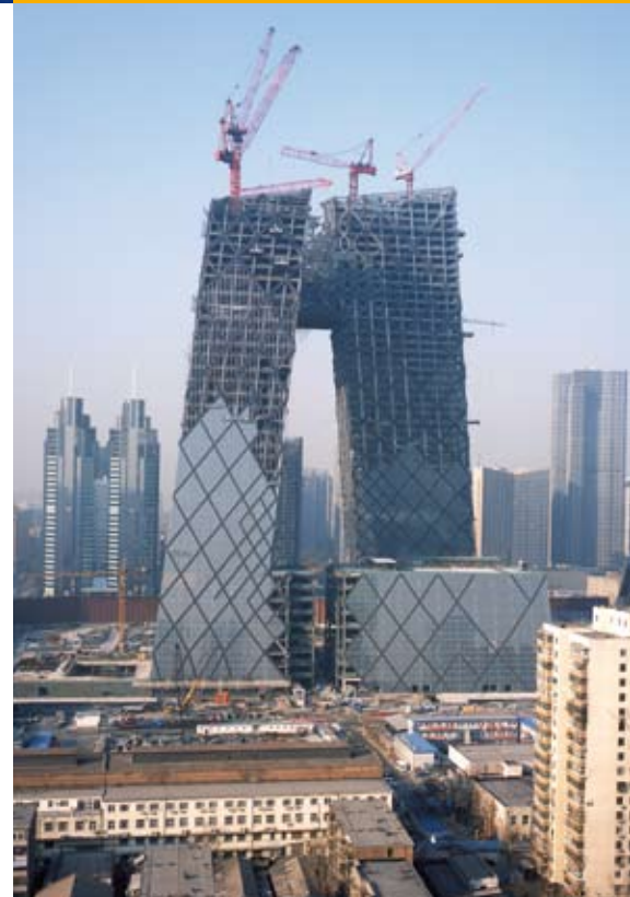
DHV played a leading role in the drawing-up of the acoustic design for Chinese State Television's new headquarters building.
