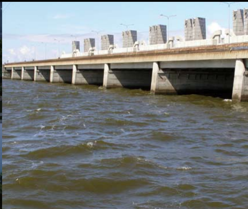
DHV was responsible for the complex hydraulic engineering for the St Petersburg Storm Barrier.
